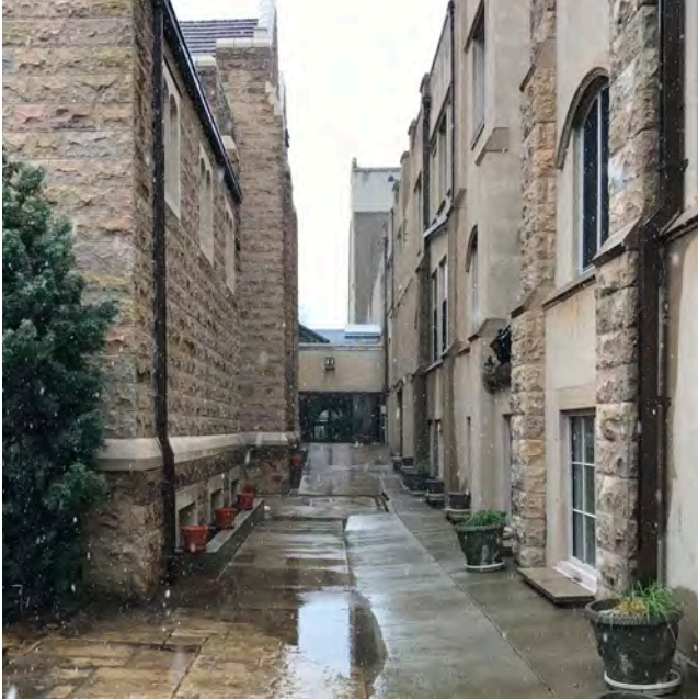
View from Eudora Street - Before
