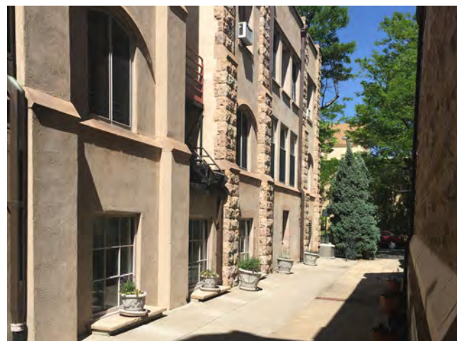
Eudora Street entry lane - Education Wing at left
