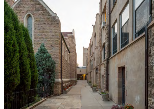
Eudora Street Entry - looking west
