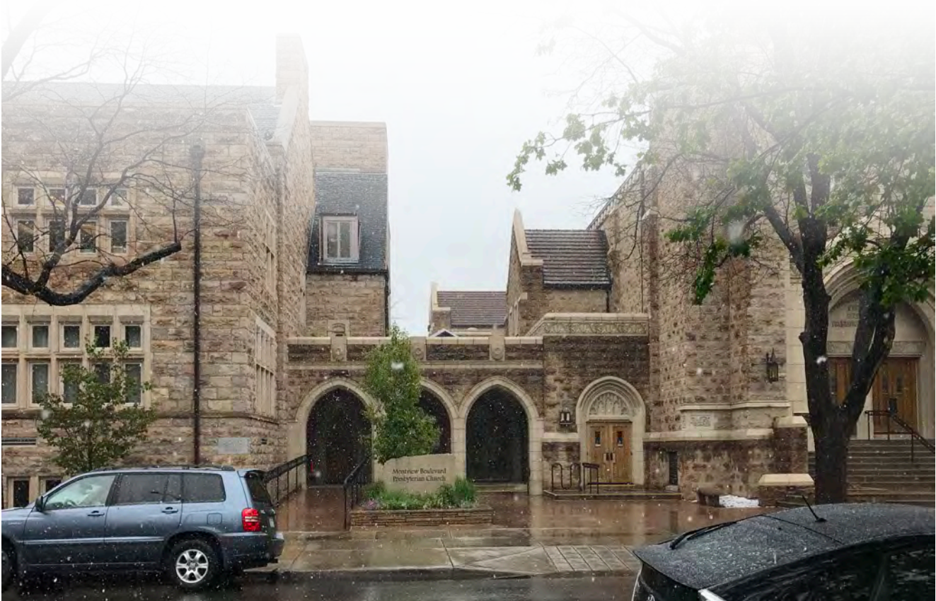
View from Dahlia Street - Before
