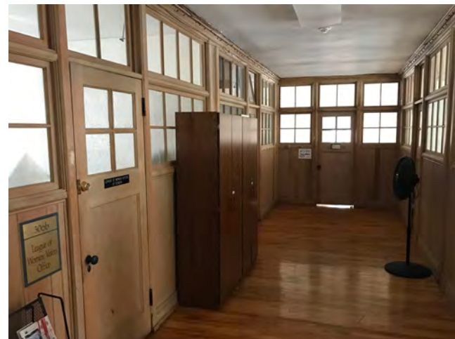
Level 2 Offices with historic partitions
